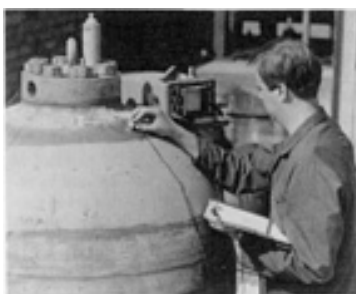
FIG. 5 ULTRASONIC EXAMINATION OF A NOZZLE WELD
