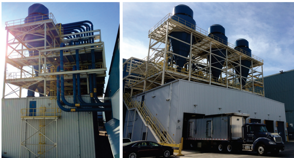
Fig. 6 — East side cyclones and sorting tubes at Dearborn Stamping Plant, September 2014. Courtesy of L. Chappuis.
